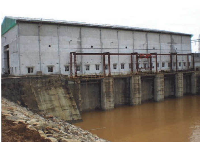
SAMAL HYDRO ELECTRIC PROJECT POWER HOUSE, KULEI VILLAGE, ANGUL
