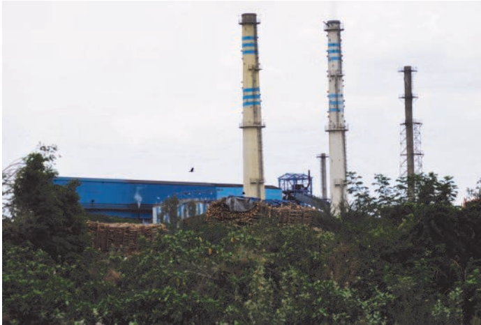
ITC FACTORY AT SARAPAKA, KHAMMAM
